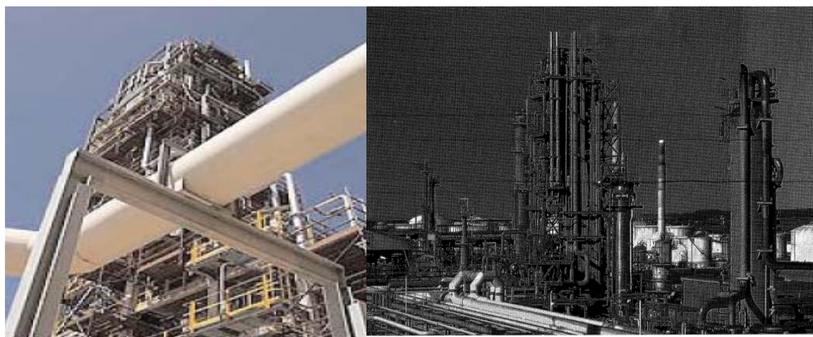
PetroSA-Statoil-Lurgi demonstration GTL plant (Photo courtesy Statoil)
