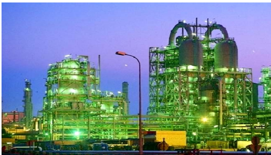
(Photo-courtesy Sasol) Sasol SAS and Synthol reactors
