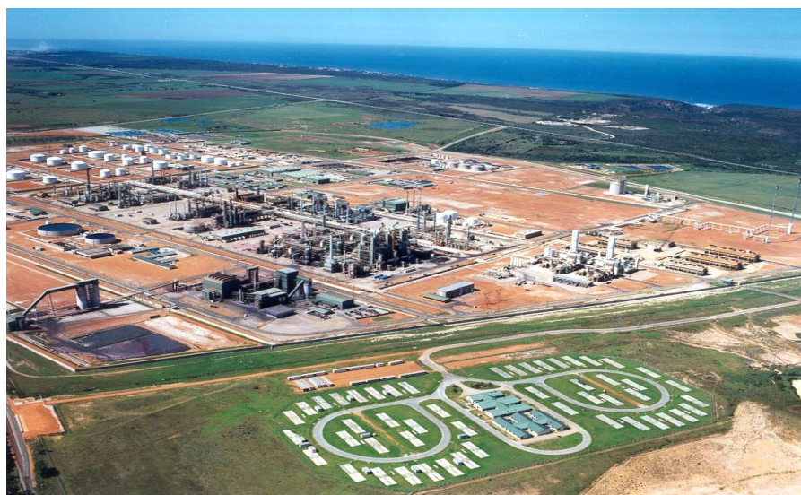
PetroSA GTL Plant Overview
