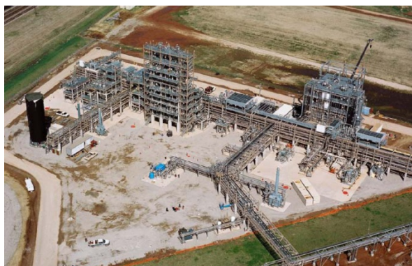
ConocoPhillips GTL Plant Picture 2003
