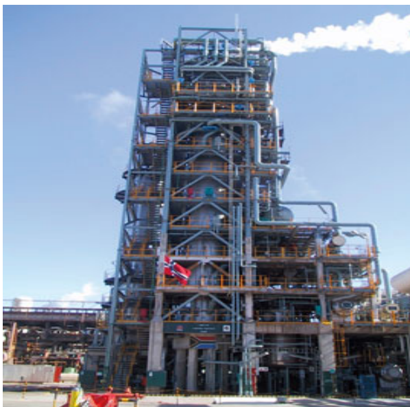
PetroSA-Statoil-Lurgi demonstration GTL plant (Photo courtesy Statoil)
