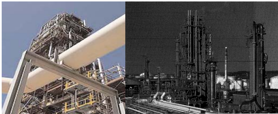
PetroSA-Statoil-Lurgi demonstration GTL plant (Photo courtesy Statoil)
