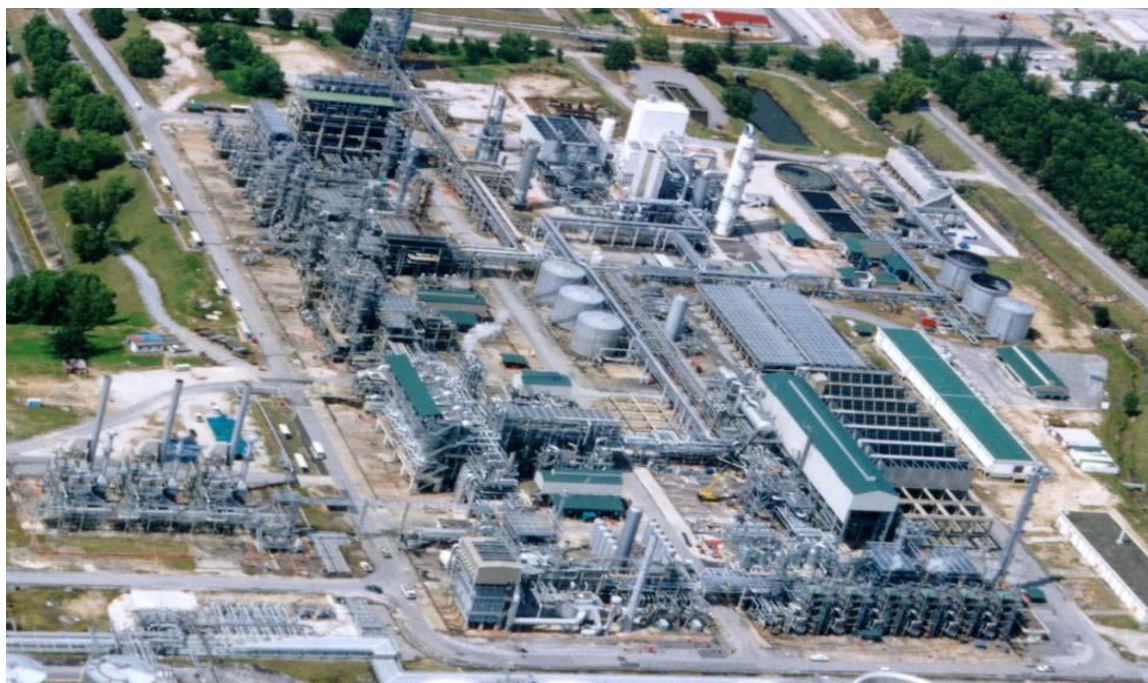
Shell Middle Distillate Synthesis Plant, Bintulu, Malaysia 2005 (photo courtesy of Shell)
