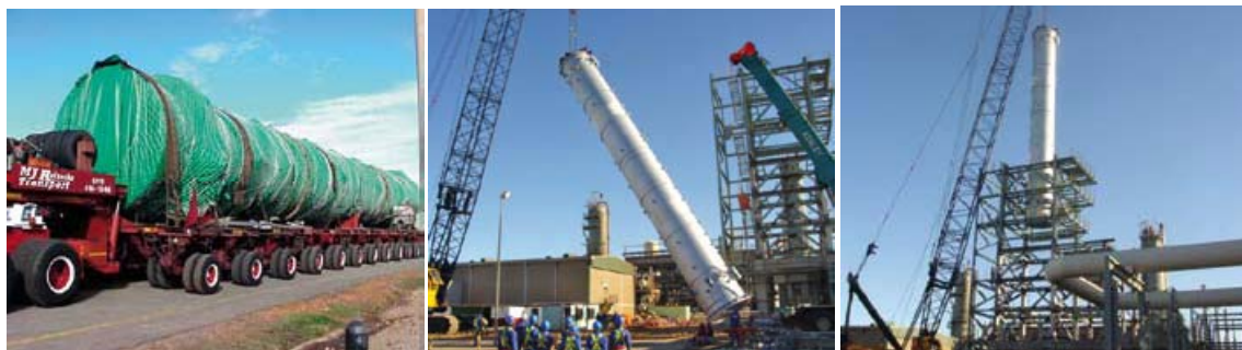
Reactor transport and installation. (Source [106] )
